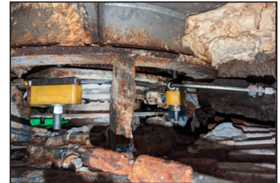
Equipment with AMPS technology installed on all four bolts.
